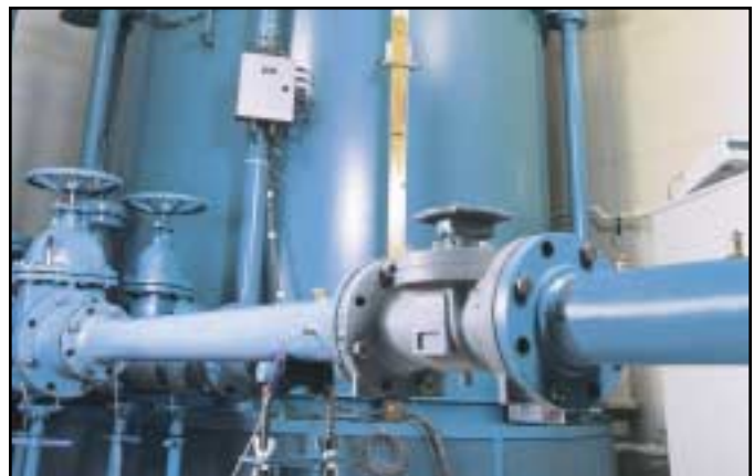
Top and Middle Photos: High pressure test facilities. Bottom Photo: Low pressure 350 ft. 3 (10M 3 ) Bell Prover.
